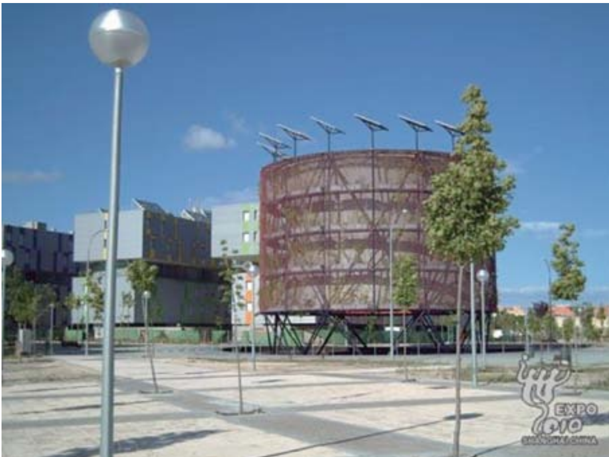
Fig. 10 The "Bamboo House" and "Air Tree" of Madrid 图10 马德里的“竹屋”和“空气树”
